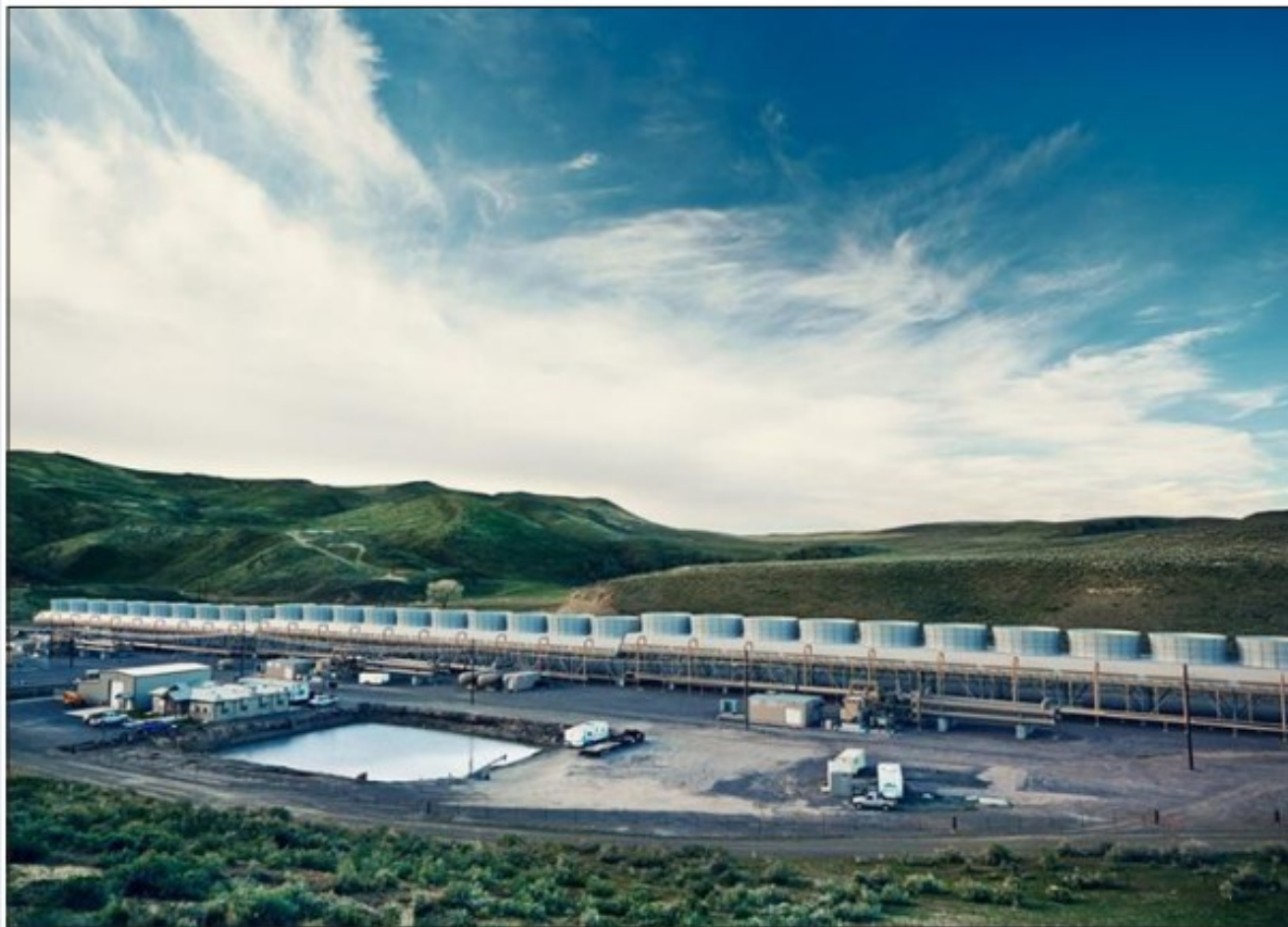
Figure 12. Neal HS 30 MW Plant. Courtesy US Geothermal.
